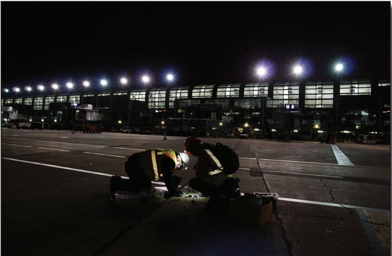
Figure 1. Students installing sensors in pavement at O'Hare International Airport
