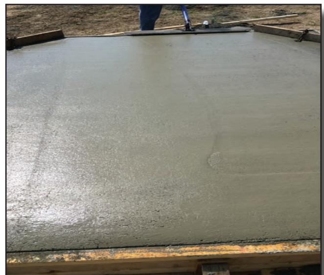
Figure 1. Mock-up slab placement with different top rebar spacing of 5x6 in. and 15x6 in. that correspond to different longitudinal rebar spacing locations along the bridge deck
