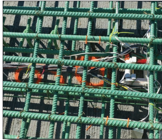
Figure 2. Sensor tower contains three humidity sensors, three thermocouples, and twelve concrete strain gages (six on tower and six adjacent to the steel rebars)
