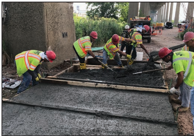
(a) Casting trial slab
