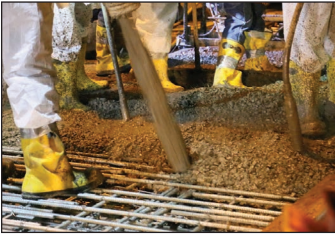
(a) Casting reconstructed bridge decks
